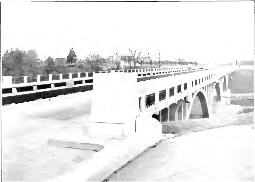
Queen Elizabeth Way — Henley Bridge
